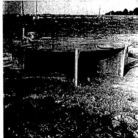
Fig. 22.2 Outlet from the gas supply duct at the release point
