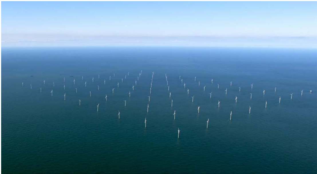
Figure 16: Horns Rev I wind farm
